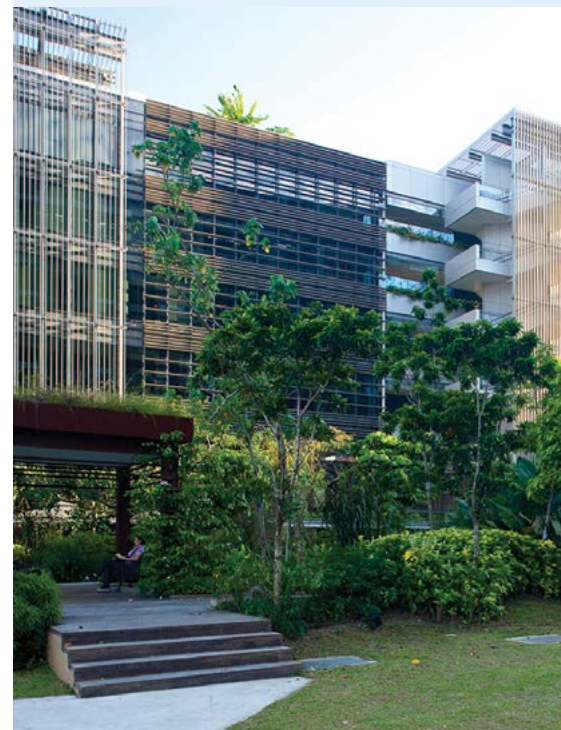
Above: The Khoo Teck Puat Hospital in Singapore, by RMJM Architects and CPG Consultants, incorporates façade solutions that allow fresh air and sunlight to increase thermal comfort. Image © Jui-Yong Sim/Flickr.
