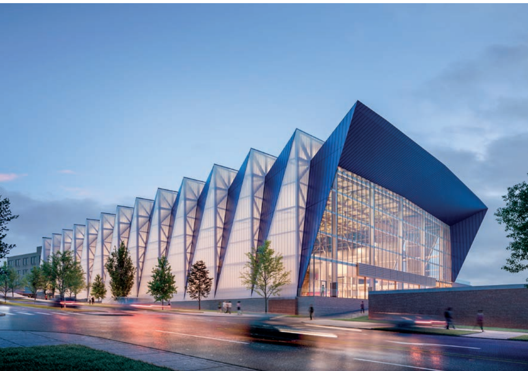
University of Cincinnati Indoor Practice Facility and Performance Center, Cincinnati
