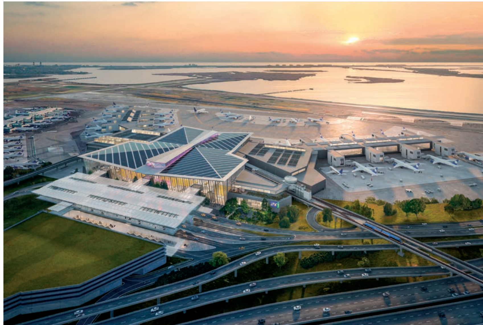
JFK New Terminal One, Queens, N.Y.
