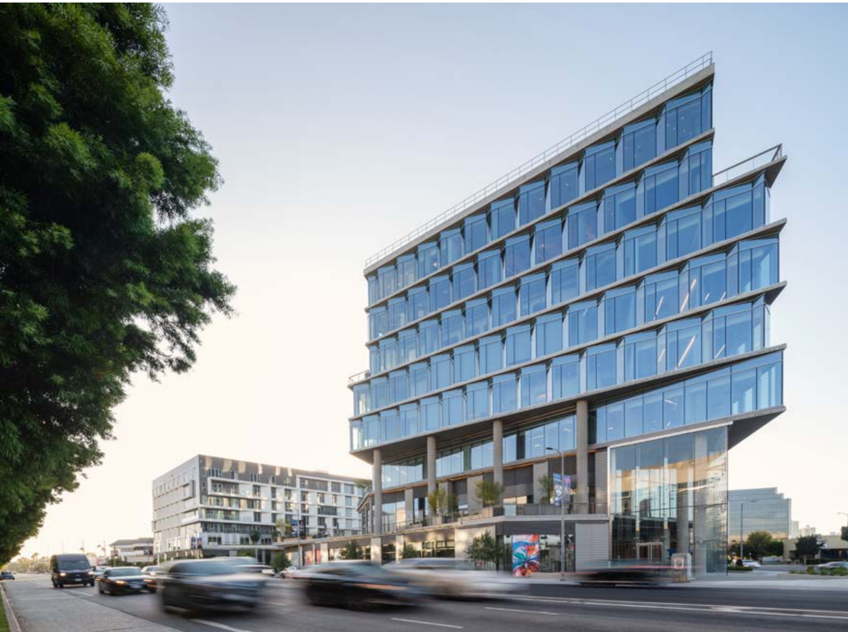
West Edge, Los Angeles Hines, Philena Properties, LLP Transit-oriented development
