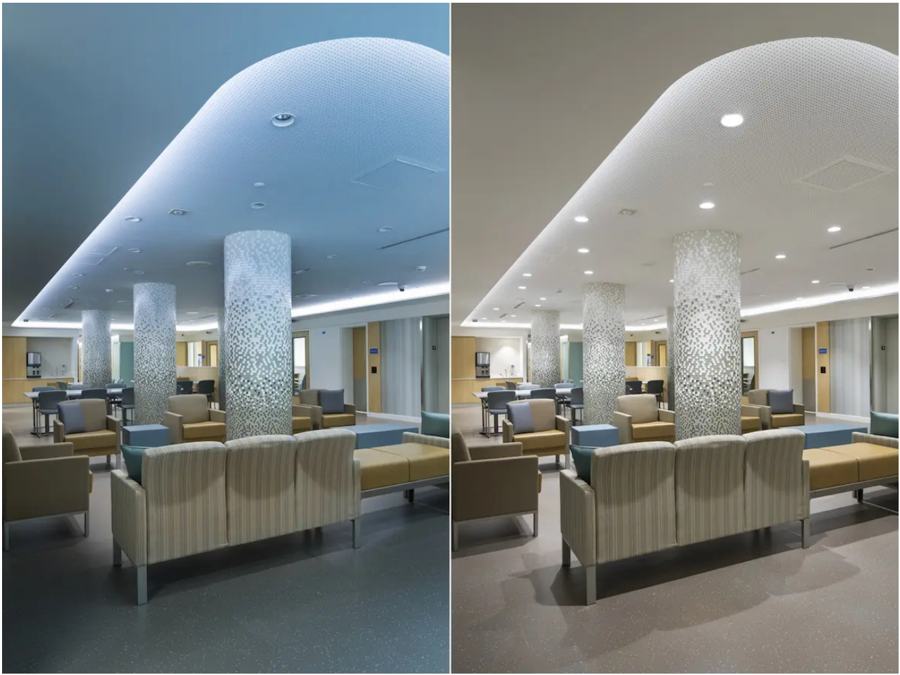
Tunable LED lighting is a perfect way to create circadian lighting. [Photo: Benjamin Benschneider Photography]
