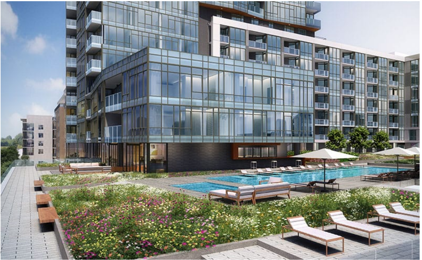
NAVA Real Estate Development's Lakehouse building in Denver incorporates extensive landscaping with the aim of creating spaces that are immersive and calming. (NAVA Real Estate Development)
