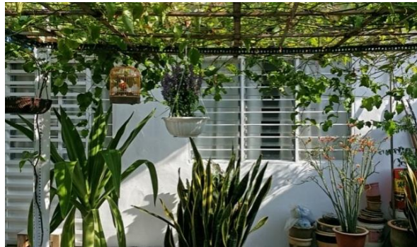
Fig. 3 Vegetated trellises provide shade for the wall of the rooms. Source: Author
