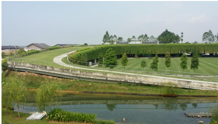
Fig. 1 Intensive vegetated roof in Malaysia. Source: Author
