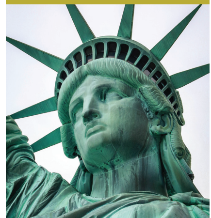
The iconic green patina on the Statue of Liberty is not original. It formed naturally over time from the same chemical process that breaks down VOCs and other noxious gasses in the atmosphere.
