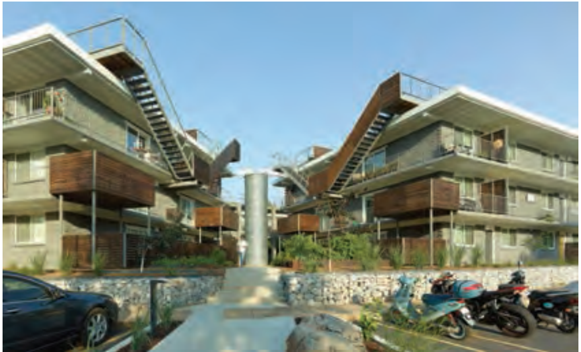
A rain garden and cistern are examples of the green infrastructure at the ECO Modern Flats in Fayetteville, Arkansas. (Timothy Hursley)
