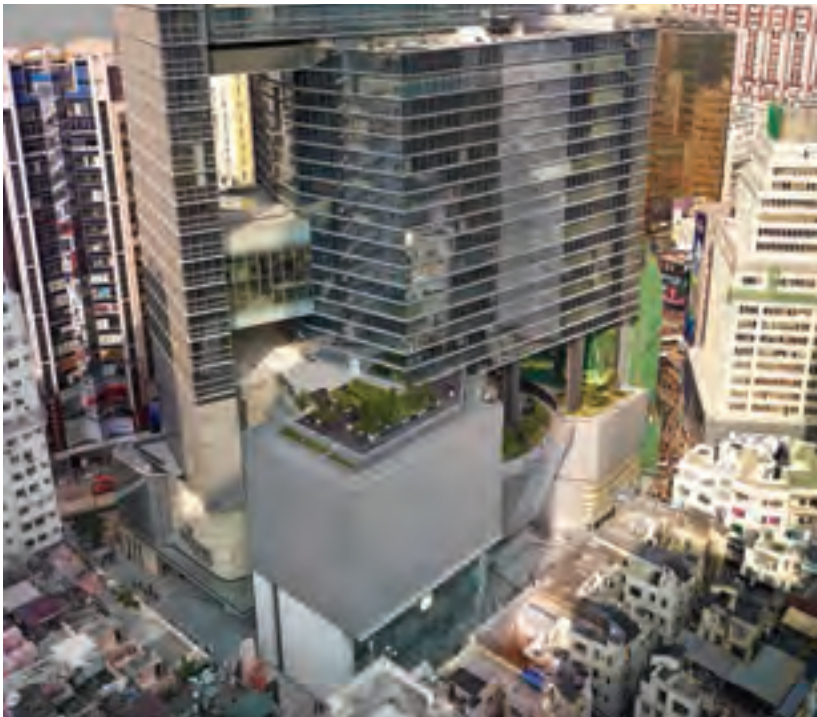
Green roof terraces at Hysan Place, a sustainable commercial building in Hong Kong, provide oases for building occupants and openings for breezes to pass through. (Grischa Rüschenndorf)
