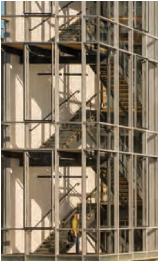
Attractive interior staircases can encourage people to take the stairs rather than the elevator. (©Nic Lehoux)
