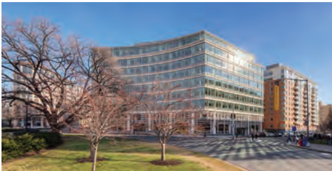
The Avenue, a mixed-use development near George Washington University in Washington, D.C., contains office, residential, and retail space, including a grocery store, a bank, and restaurants. (Kevin Weber)
